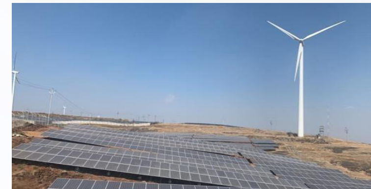
Solar Power Plant Ahmednagar, Maharashtra (5.2 MW)
