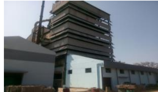
Unit 3 - New Reactive Dyes Plant
