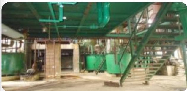
Sulphuric Acid Plant
