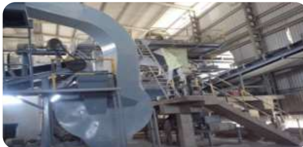
Unit 2– Granulation Plant
