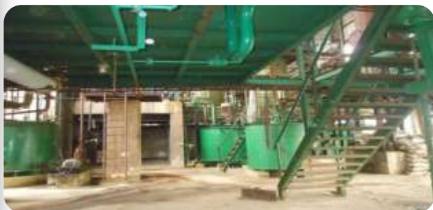
Sulphuric Acid Plant
