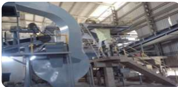
Unit 2– Granulation Plant
