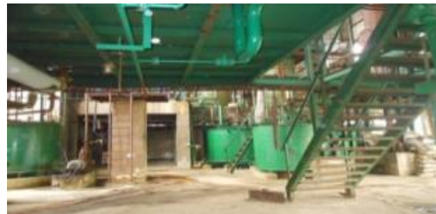
Sulphuric Acid Plant
