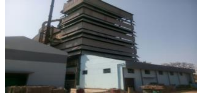
New Reactive Dyes Plant Unit 3
