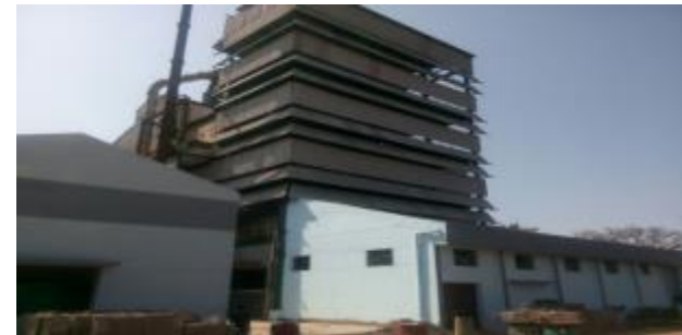
Unit 3 - New Reactive Dyes Plant
