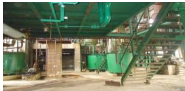
Sulphuric Acid Plant
